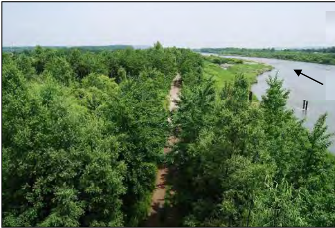
⑤十勝大橋下流左岸(築堤側)
